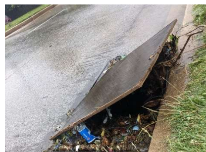
Blocked storm drain during flooding on Hillen Road on June 10, 2021.
