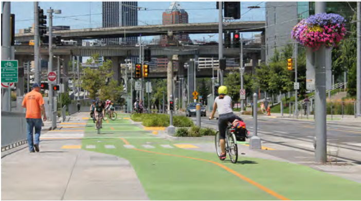
This design highlights cycle and pedestrian lanes that are integrated with stormwater management practices (bioretention) along a major roadway. Portland, OR
