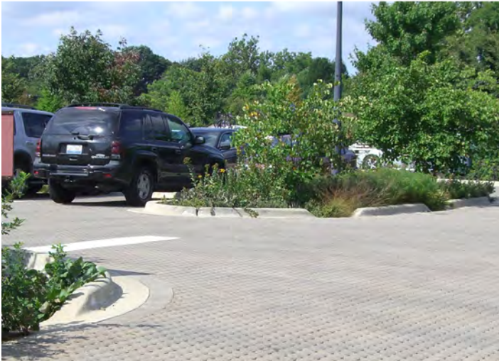
Parking can include permeable paver, integrated bioretention and increased tree canopy. Chicago, IL
