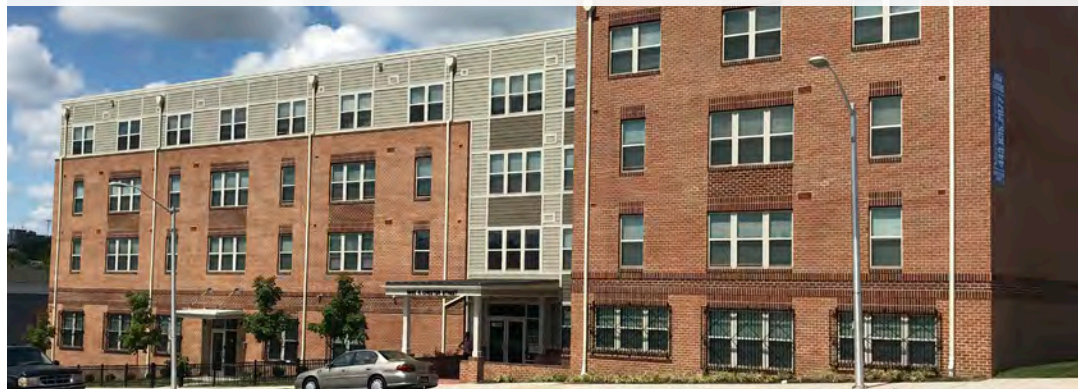
The Mary Harvin Senior Center is part of a revitalization strategy in Broadway East.
