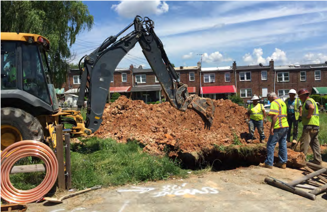
Water line installation in the Berea neighborhood, expands access to water.
