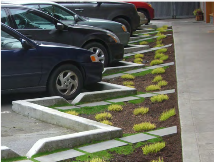
Bioretention can also be designed as smaller integrated planters to collect and treat water in smaller parking areas. Portland, OR.
