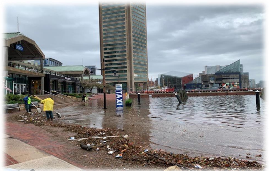
Figure 12: Flooding along Baltimore's Inner Harbor promenade in April 2020.
