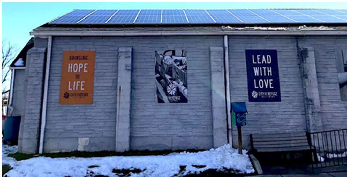
City of Refuge, a Resiliency Hub in the Brooklyn neighborhood of South Baltimore, received solar power and battery storage through the Baltimore City Community Resiliency Hub Program. Funding was made possible through a grant from the Maryland Energy Administration and a partnership with Groundswell, A.F. Mensah, and Suncatch Energy. – photo by Aubrey Germ, BoS Staff
