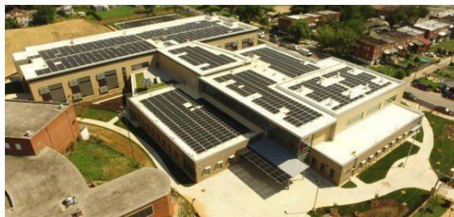
The newly-constructed Graceland Park-O'Donnell Heights Elementary School - photo courtesy of Baltimore City Public Schools
