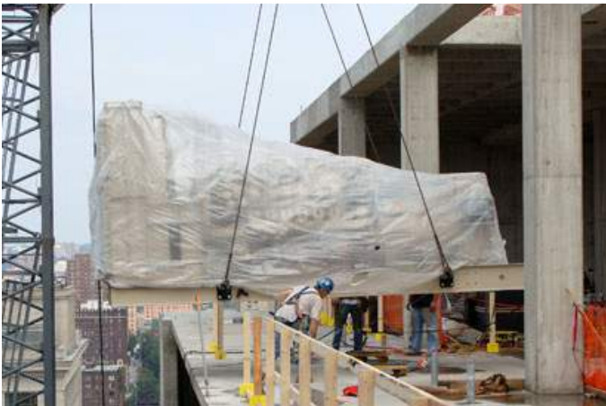
Generator Installation at Mercy Hospital Source: Curtis Engine
