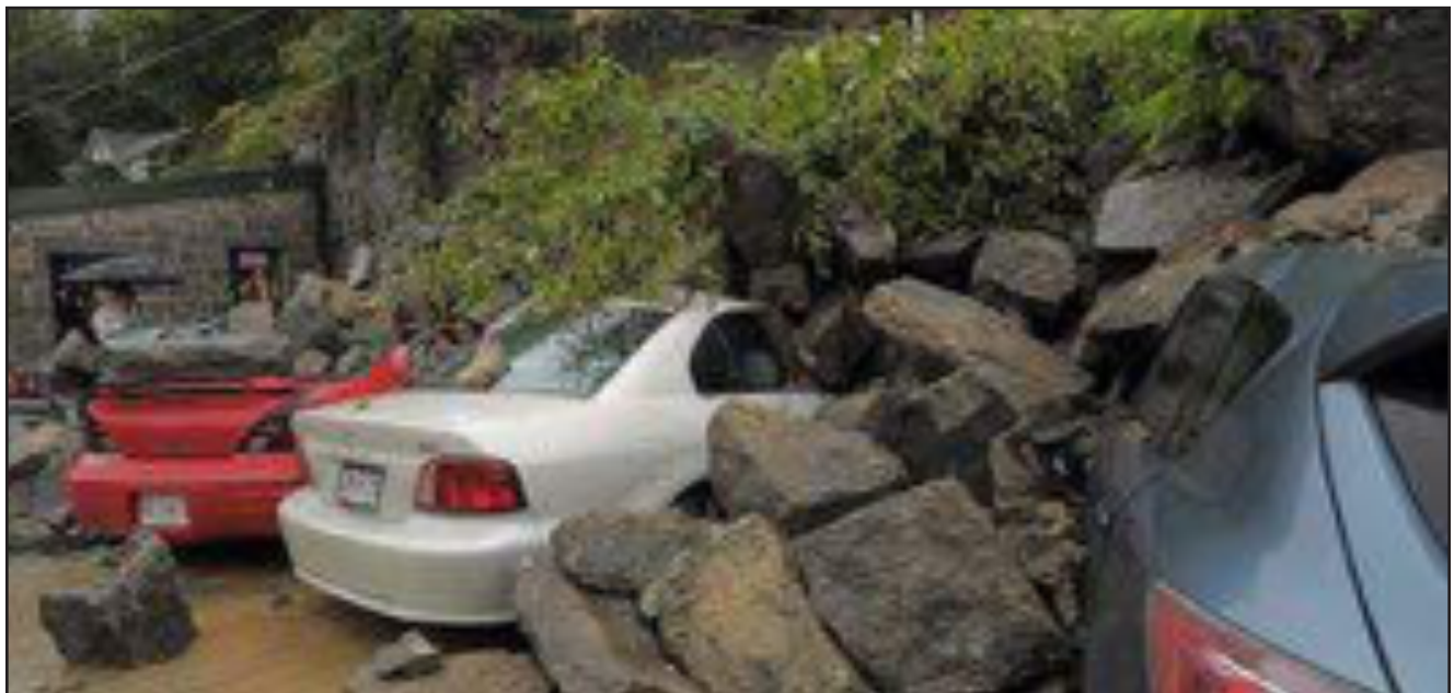
A retaining wall in Ellicott City, MD collapses following heavy rains
